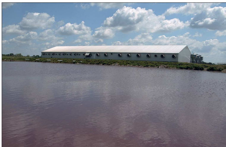
Liquefied manure flushed from the main hog barn at a farm in Fillmore, Ind., is stored in a large “lagoon” until it can be sprayed on fields as fertilizer. Pollution occurs when lagoons leak into streams or groundwater, or farmers apply manure to land faster than plants can take up its nitrogen and phosphorus, leaving excess that washes out of soils.
