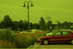
Bioswale and Porous Pavement
