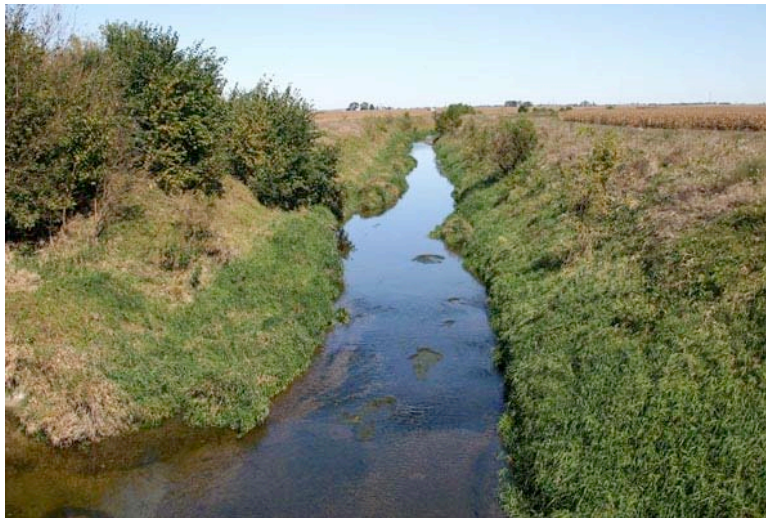
Figure 25 – Example of stabilized two-stage channel design
