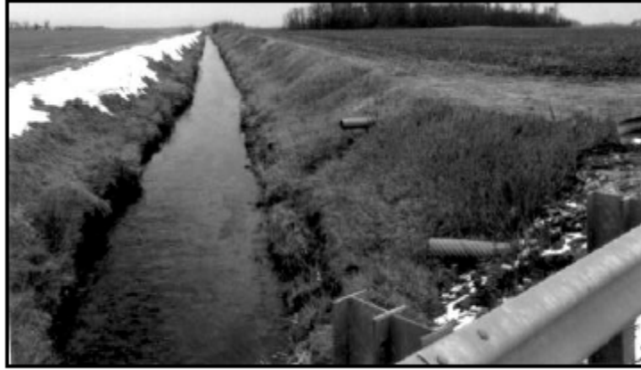
Figure 17 – Example of an outlet extension (Image from Indiana Drainage Handbook and courtesy of Tipton County)
