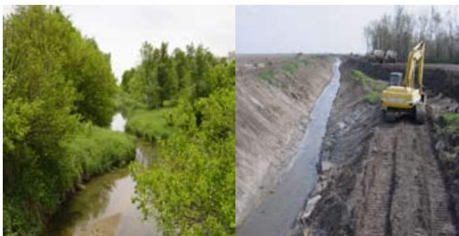
The photos above show the Spoon River before and after being dredged for drainage maintenance.
