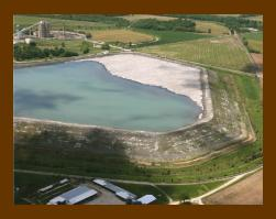
Most coal slurry pits in Illinois do not have protective liners. Because so many lack this basic environmental protection, harmul pollution from coal waste has polluted local groundwater and streams across Illinois. Discharges from coal slurry pits also add pollution to rivers and streams.
