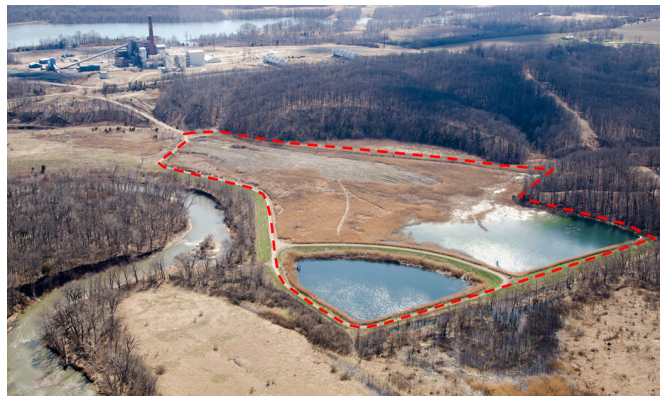
A 40-acre coal ash impoundment at the Vermilion Power Station is outlined in red. It is one of three at the site. The power plant in the background provides a sense of scale.
