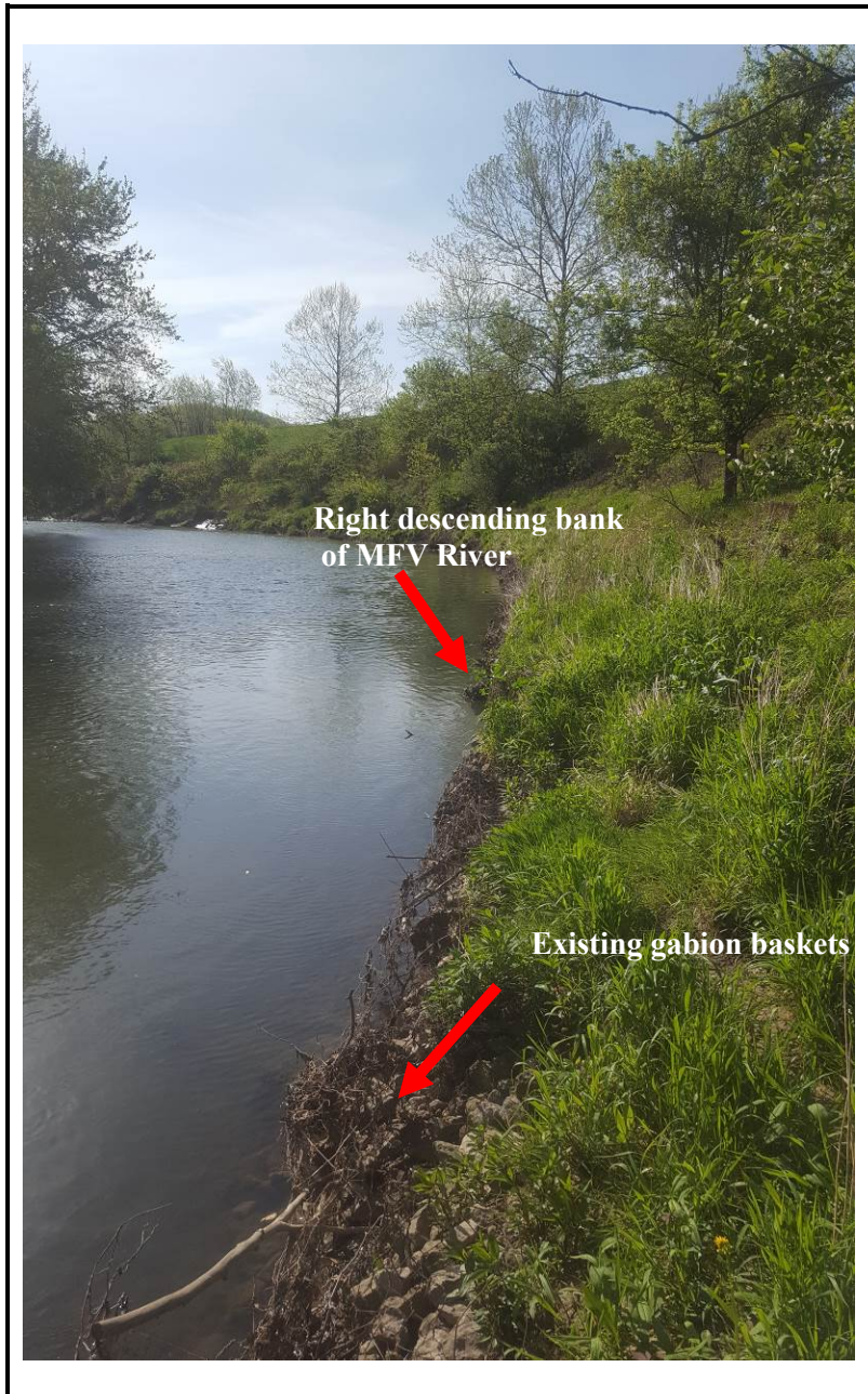
Photo 4. Photo along the right descending bank of the river showing the existing gabion baskets, facing downstream south (4-26-17)
