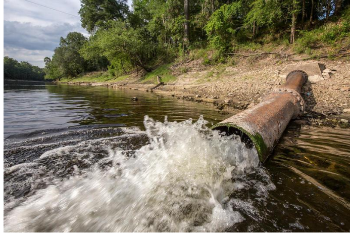
In Live Oak, Florida, wastewater pours from a Pilgrim's Pride meat processing plant into the Suwannee River
