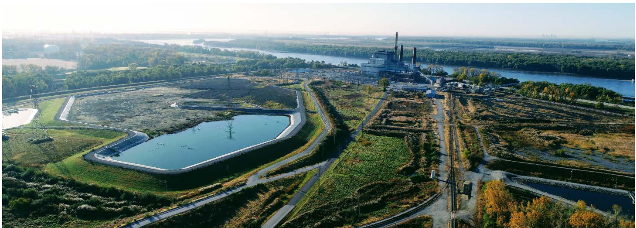
The Wood River power plant near Alton IL. Multiple coal ash ponds are pictured.
